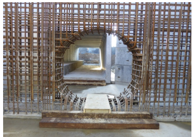
Internal view of control structure
