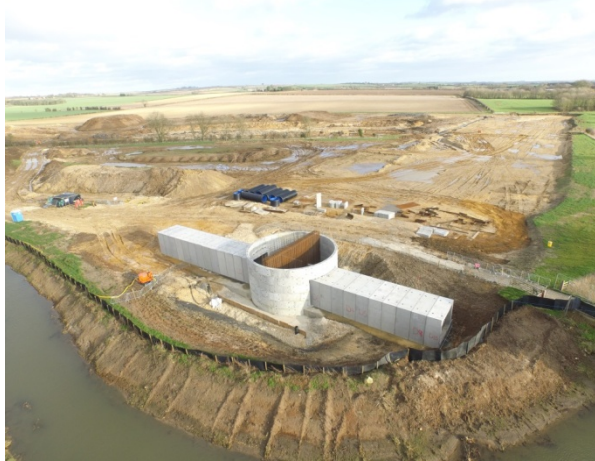
Arial view of control structure
